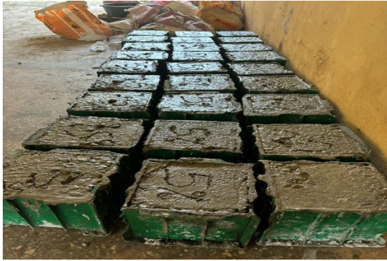
Figure 3: Concrete Placed in Moulds
